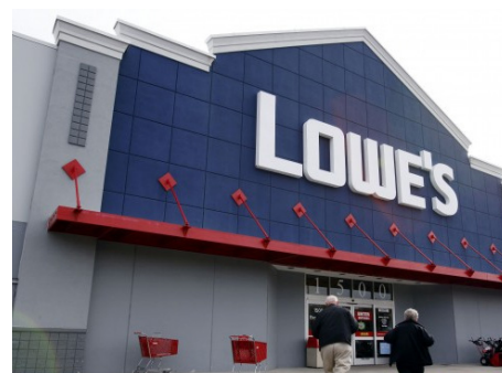
Home Improvement Center Example: Lowe's Avg. Store SF: 116,000 Site Size: 10-12 Acres
