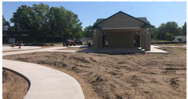
ABOVE: MEMORIAL PARK CONSTRUCTION PHOTOS TAKEN AUGUST 2021.
