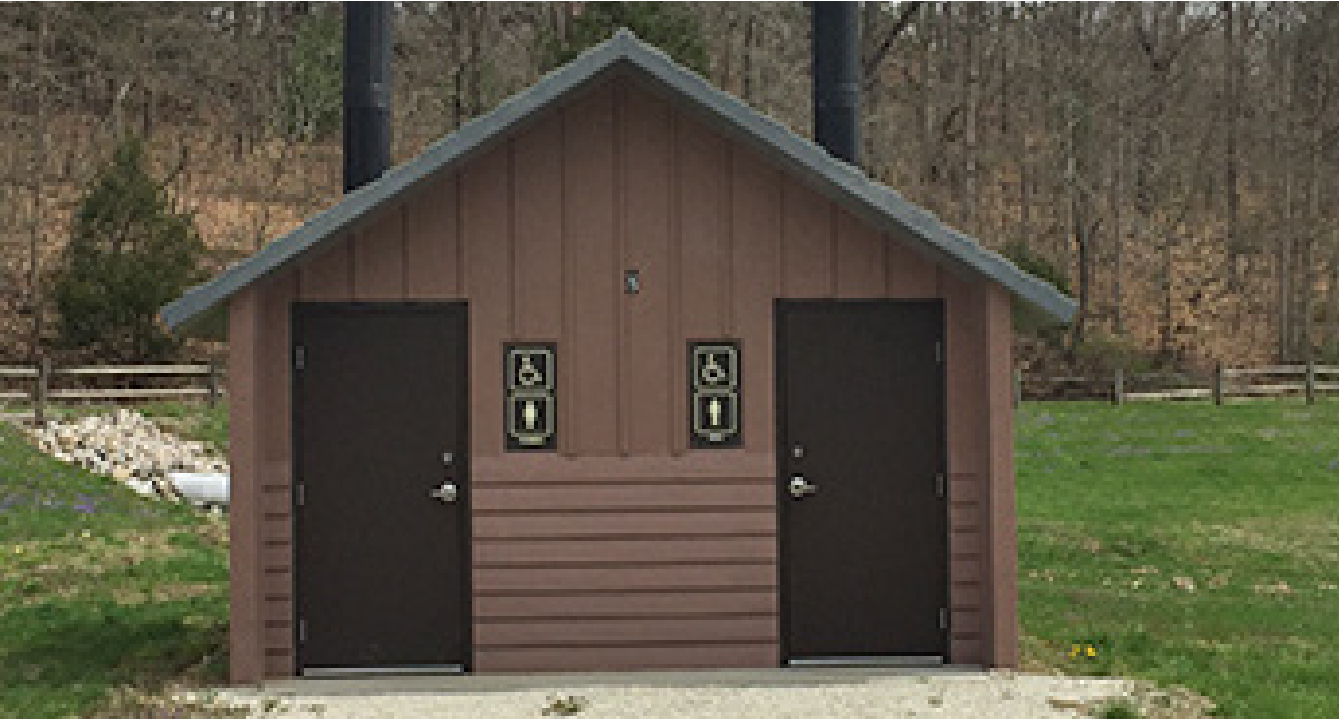
Restroom Building Form Liner
