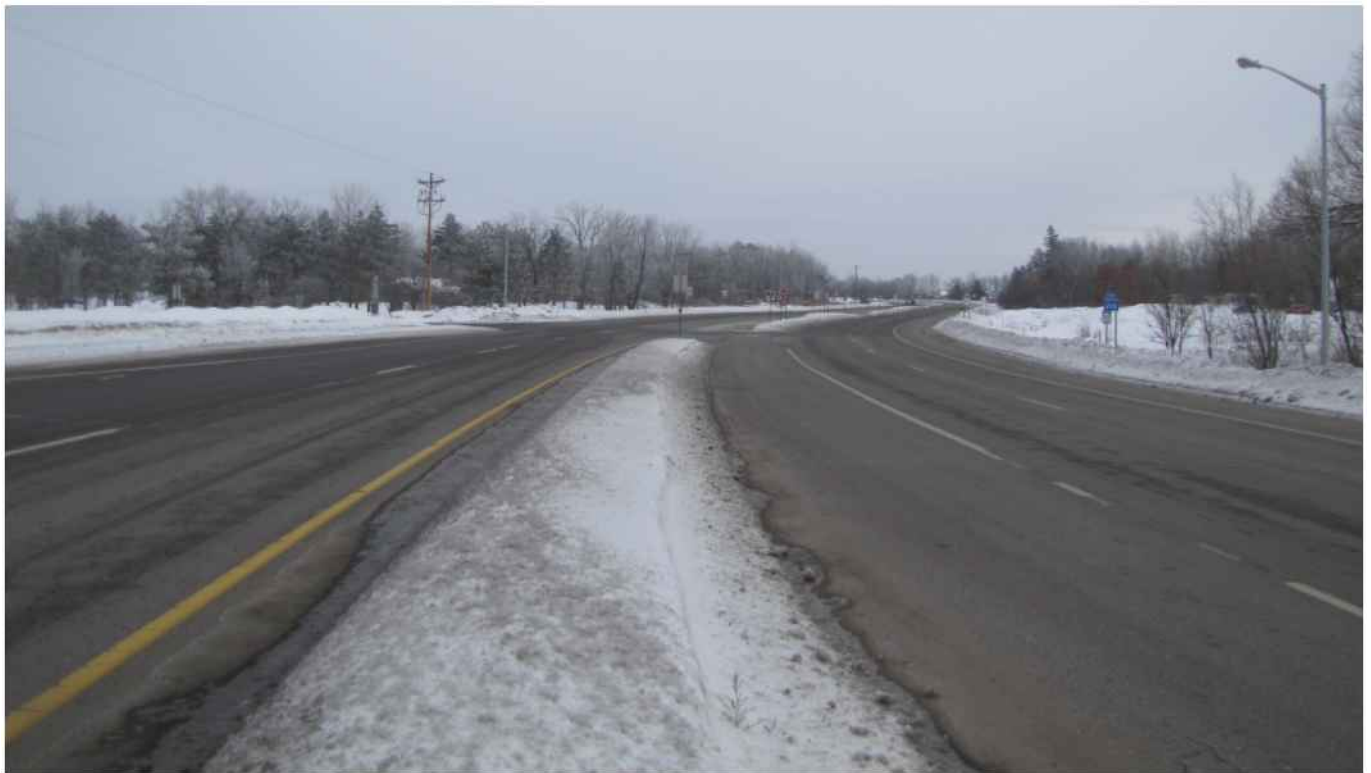
VIEW LOOKING EAST ALONG HIGHWAY 210 FROM MEDIAN WEST OF LUM PARK ROAD
