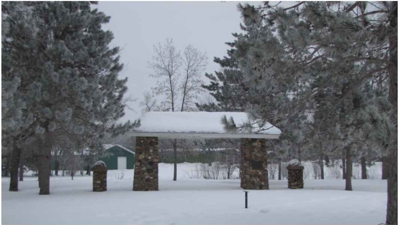
ORIGINAL STONE MASONRY ENTRANCE TO LUM PARK
