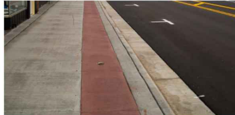
Proposed integral colored concrete along sidewalk
