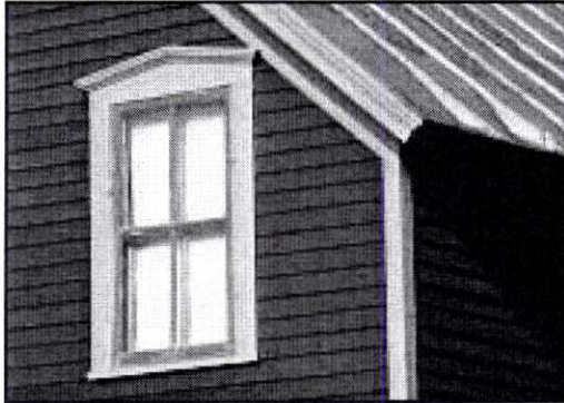
Narrow lap siding is common in older houses.
