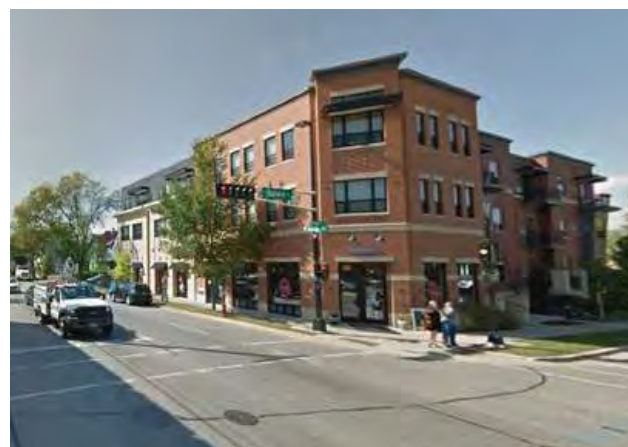
Mixed use building 1252 Williamson Street Madison, WI
