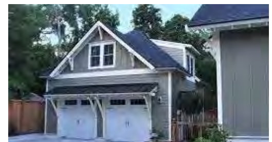
Attached to Accessory Structure
