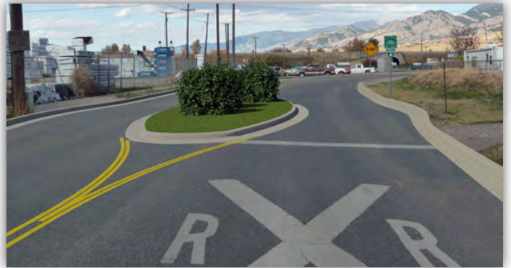
Roadway project – After
