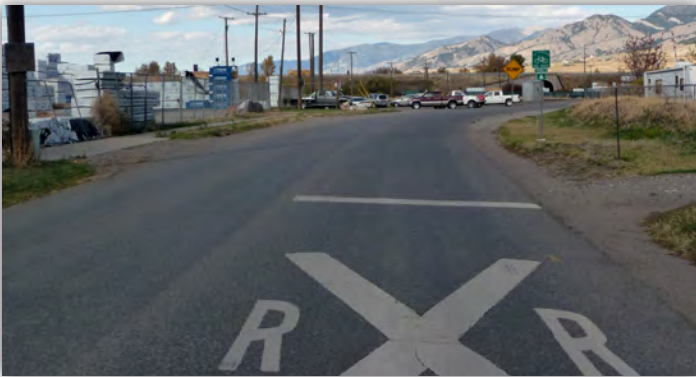
Roadway project – Before
