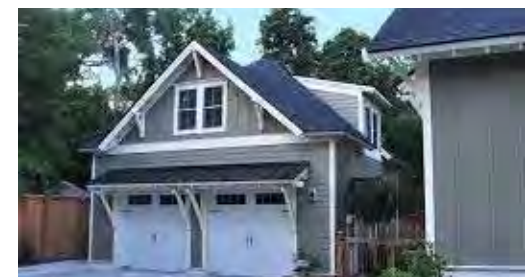
Attached to Accessory Structure
