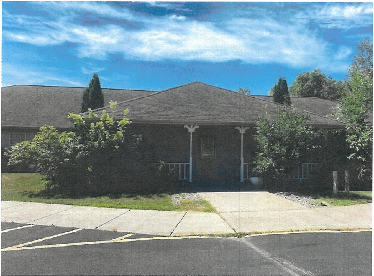
Front of Building 1
