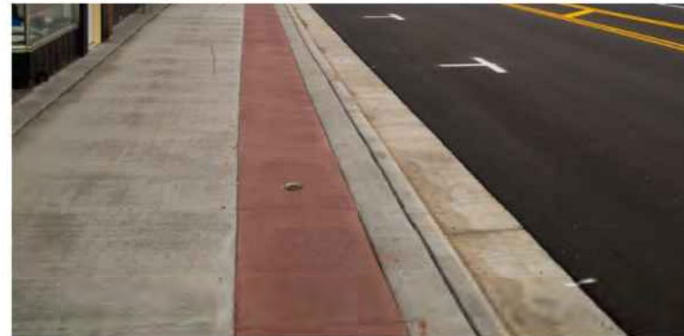
Proposed integral colored concrete along sidewalk
