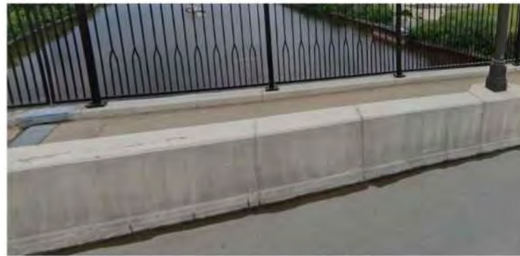
Concrete Barrier between sidewalk and traffic lanes on river bridge
