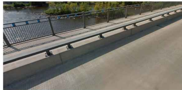
Concrete barrier between sidewalk and traffic lanes on river bridge with tube railing
