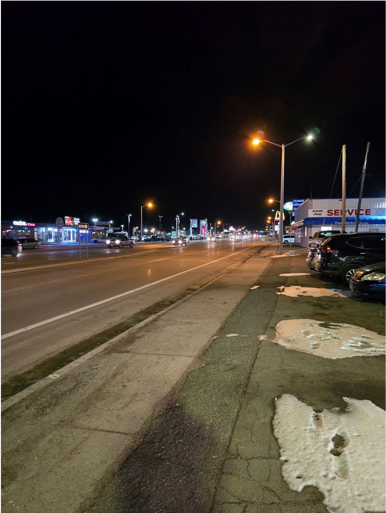
Central Brainerd Lighting – 2 lights per intersection, staggered spacing
