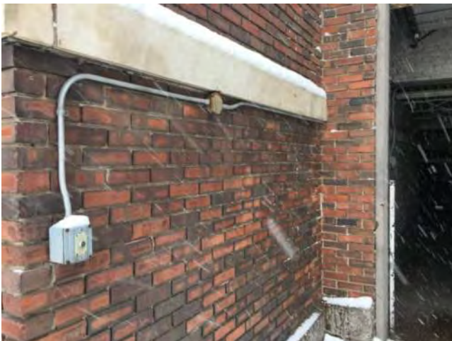
Conduit and Boxes are not Weather Proof
