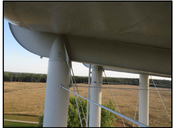
Tank Bowl I-Beam Supports
