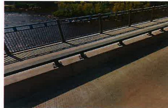
Concrete barrier between sidewalk and traffic lanes on river bridge parapet.
