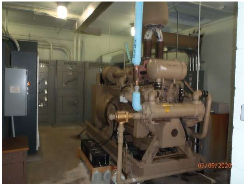
Generator on first floor of main lift stion
