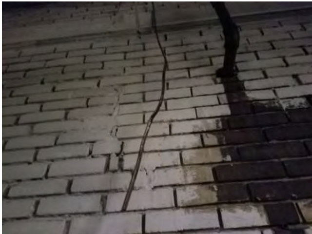
Antenna Cables run thru Garage Needs to be Strapped and rerouted
