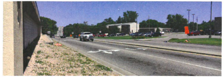
Pedestrian accommodations are not present along the CSAH 20 (NW 4 th Street) corridor.
