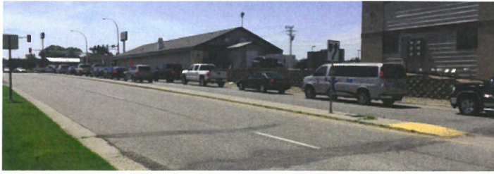
Current back-ups at Washington Street (TH 210) impact the safety and mobility of the corridor.
