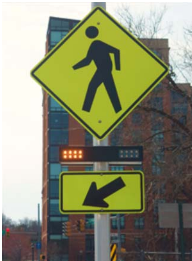
Rapid Flashing Rectangular Beacon
