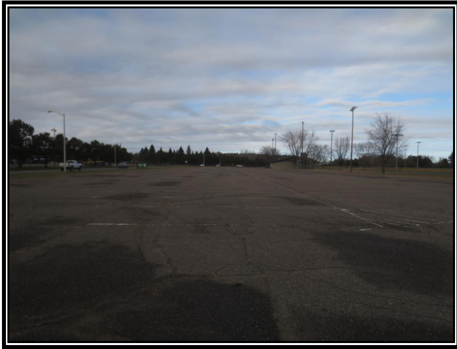
Northerly View of Parking Lot
