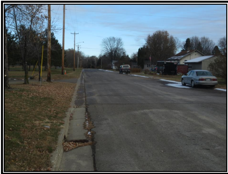
Easterly View of Q Street NE
