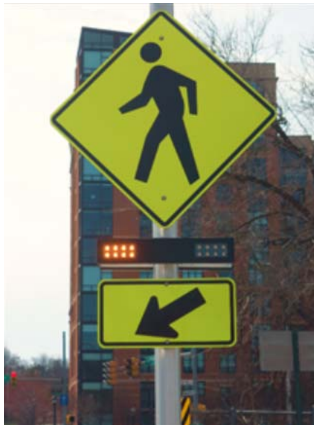
Rapid Flashing Rectangular Beacon
