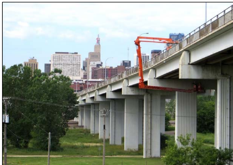
Figure 2.1: WSB PM and Lead Bridge Inspector Daniel Flittie inspecting Br 62080.
