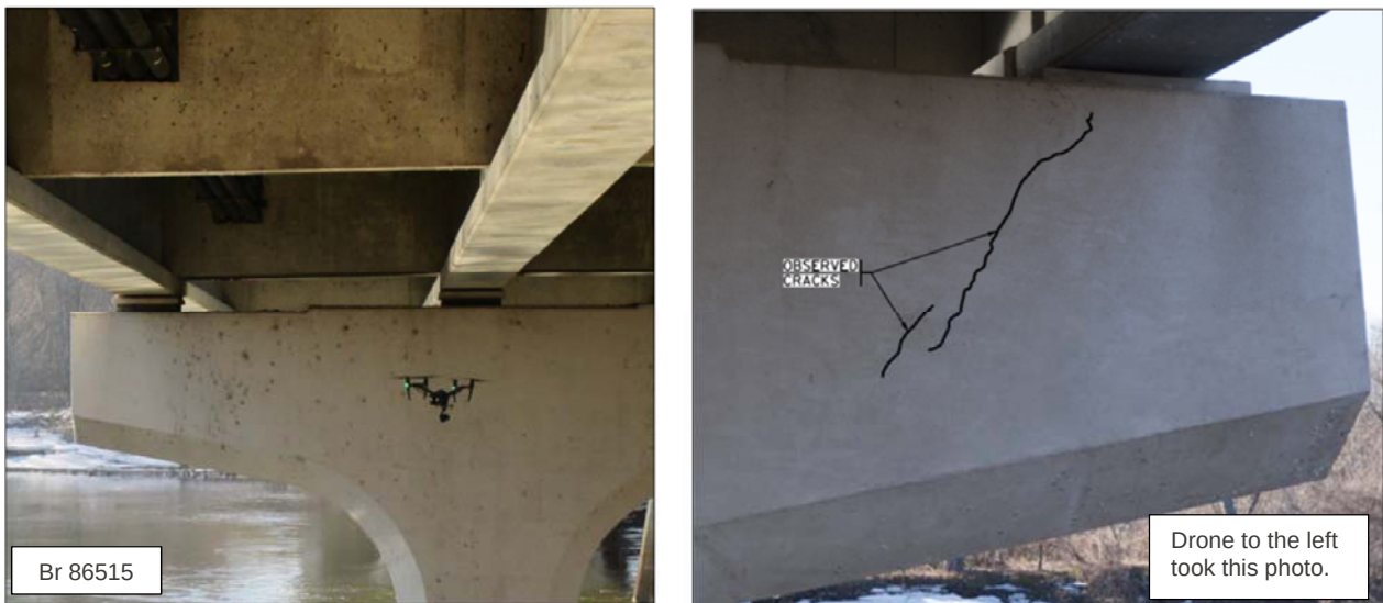
Figure 2.2: Bridge 86515, Special Drone Inspection
