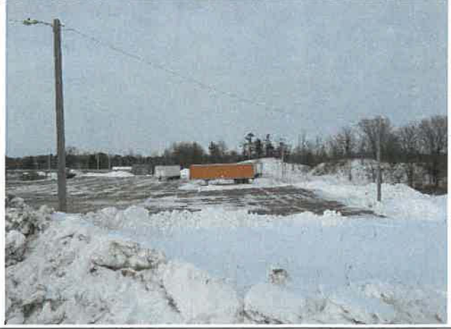
Photo 8: View of parking lot encroachment along subject W lot line; looking N from SW corner of N'y Tract
