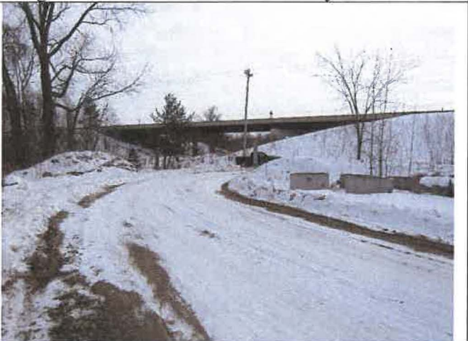
Photo 6: View of driveway TE area at E end of N'ly TE area; looking SE from N end of TE toward TH 25 bridge
