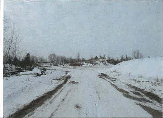
Photo 7: Interior view of subject's Northerly Tract; looking NW from E end of northerly TE area
