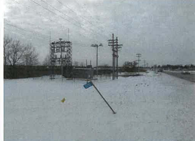
Photo 9: View of subject's S'ly Tract; looking W along TH 25 at entrance to electric substation on property
