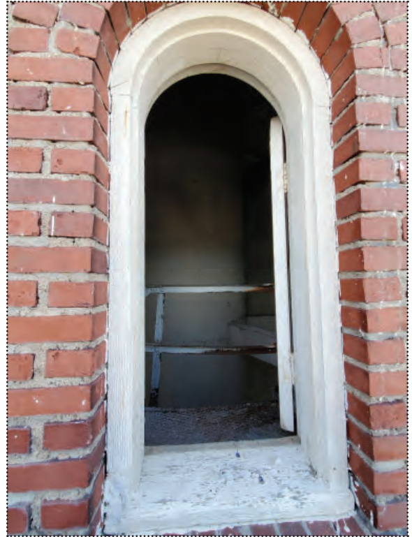
15) Window 01 from exterior stairs, 2020
