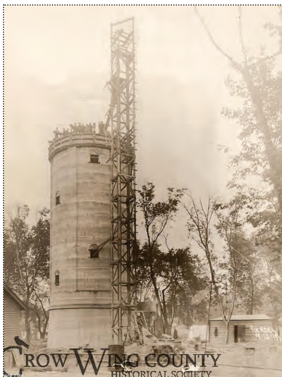
1) Water tower under construction c. 1919
