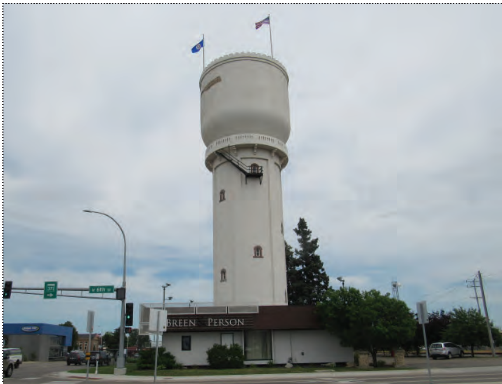
5) Looking east. Note modern exterior stairs, modern addition in the foreground, 2020
