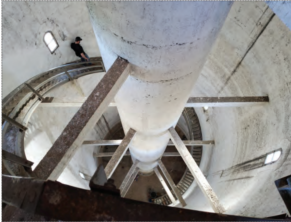
11) Looking down at stairs from near the top of the shaft stairs, 2020
