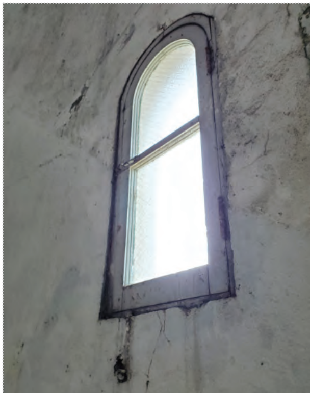
19) Window 05. Typical interior window conditions, 2020
