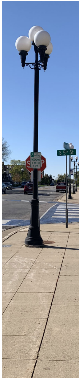
Laurel Street and Downtown Decorative Street Light (Current)
