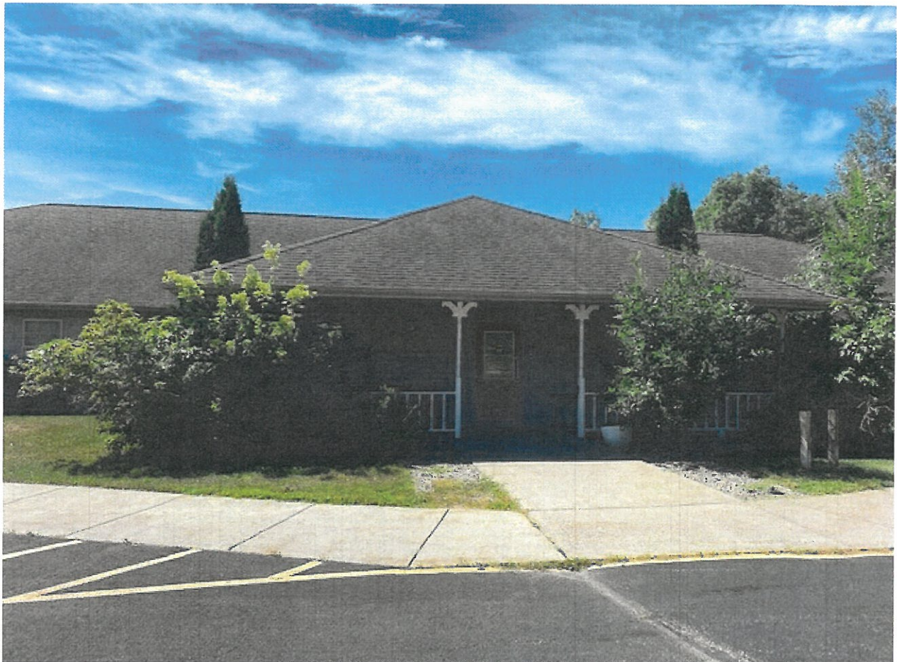
Front of Building 1
