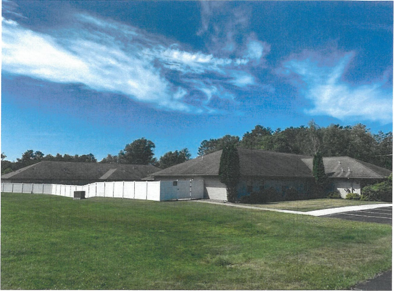
Side of building 1 with fence and building 2 in the background.
