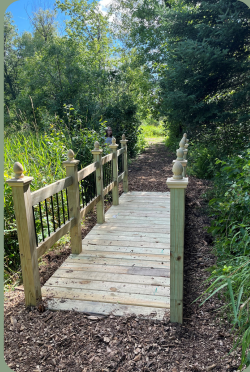
Installing footbridges and lighting for safer trails.
