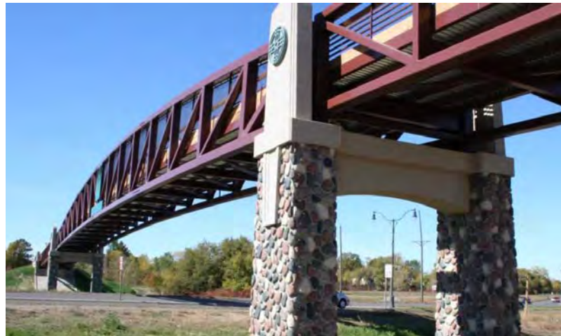
Example Bridge on Paul Bunyan State Trail
