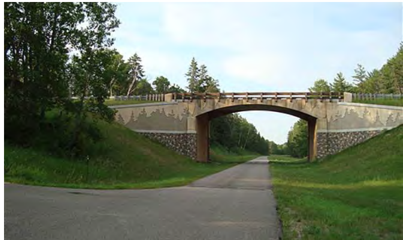
Example Bridge on Paul Bunyan State Trail
