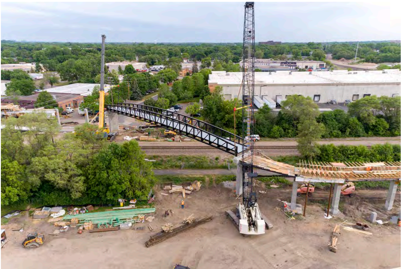
Installation of 200-foot long truss main span over BNSF track for Dakota-Edgewood Trail Bridge.
