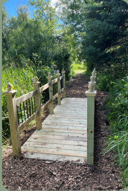
Installing footbridges and lighting for safer trails.
