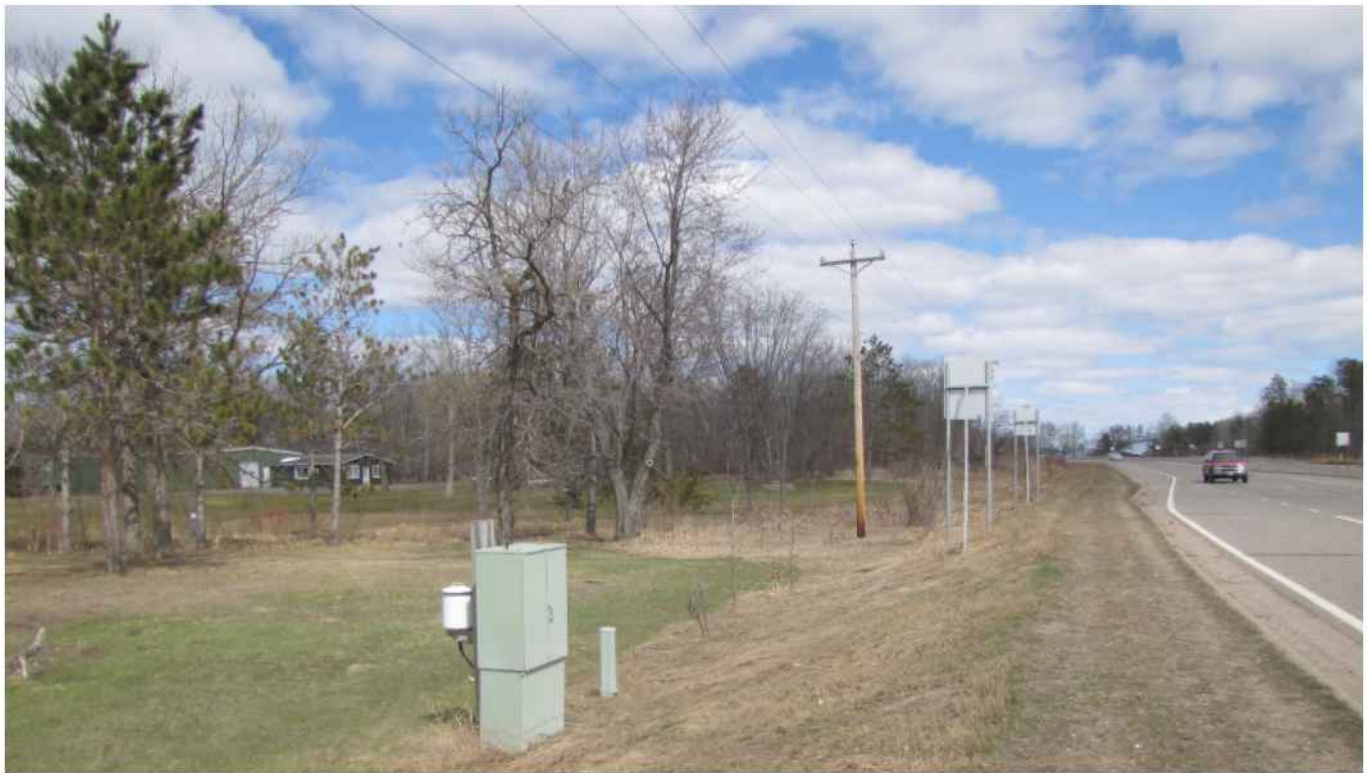
VIEW OF OVERHEAD POWER ALONG NORTH SIDE OF HIGHWAY 210 AND SOUTH SIDE OF LUM PARK
