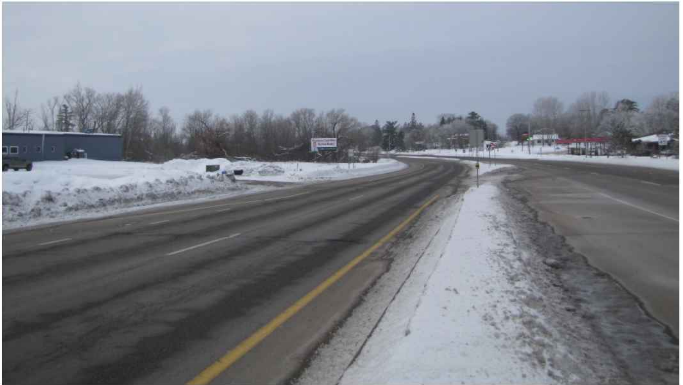
VIEW LOOKING WEST ALONG HIGHWAY 210 FROM MEDIAN AT LAURIAN LANE
