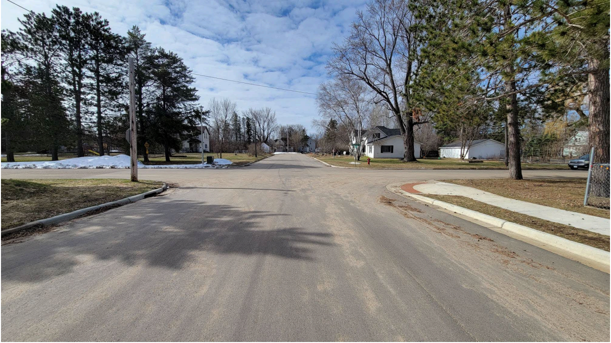
On 15 th Street SE - Looking South
