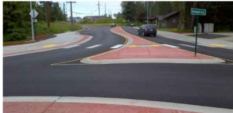
Proposed integral colored concrete in medians
