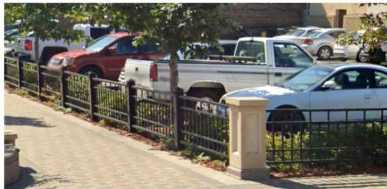
Parking lot fence
