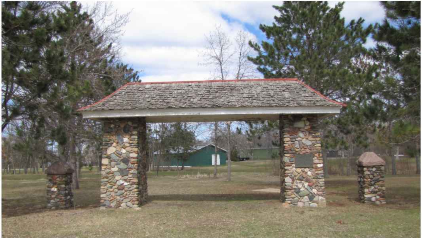
ORIGINAL STONE MASONRY ENTRANCE TO LUM PARK
