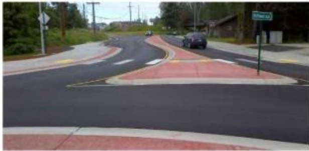
Proposed integral colored concrete in medians
